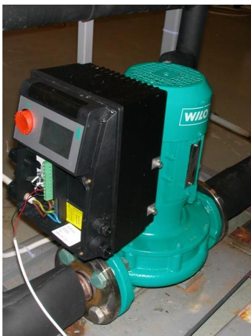
Figure 2-2 The new and smaller sized central pump.
