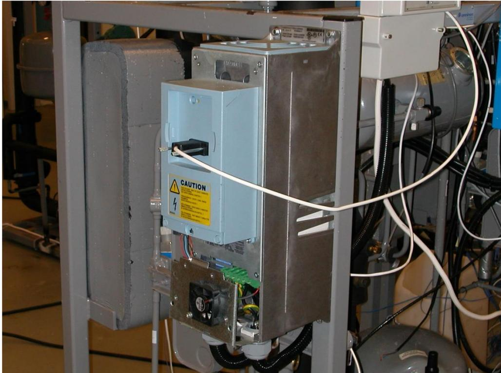
Figure 2-3 Frequency controller for the compressor control
