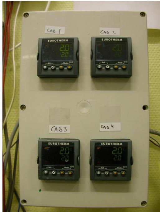
Figure 2-5 PID controllers of decentralized pumps.
