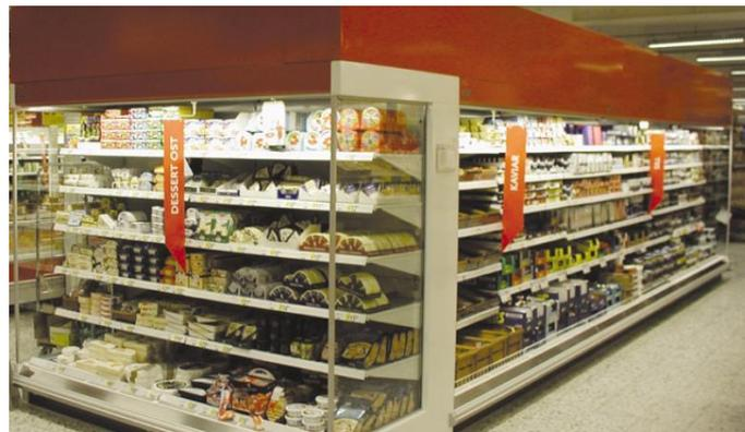
**Figure 1.** A common type of display cabinet with an indirect refrigeration system.
