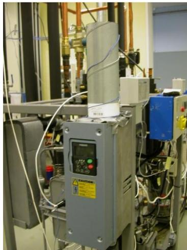
Figure 4 The frequency controller mounted with the thermocouple at the air outlet.
